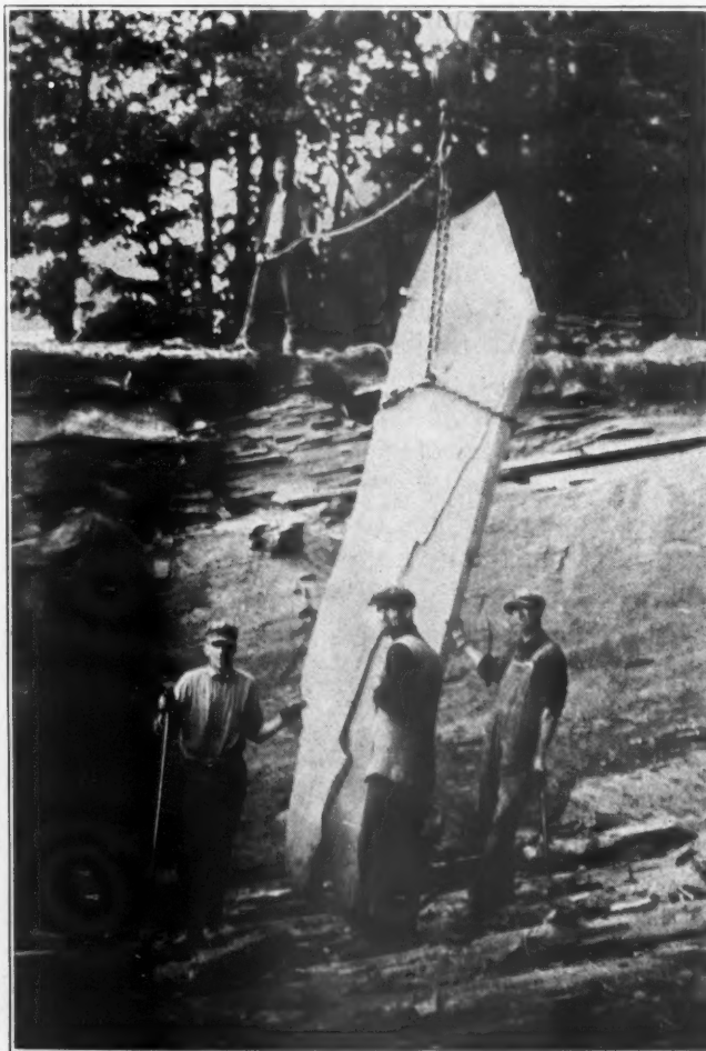
Hoisting a Large Piece of Rock from the Quarry
